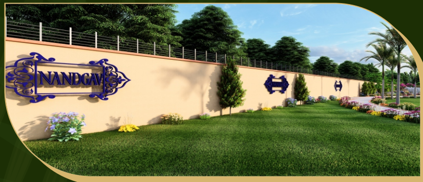
Outer Boundary with Wire Fencing
